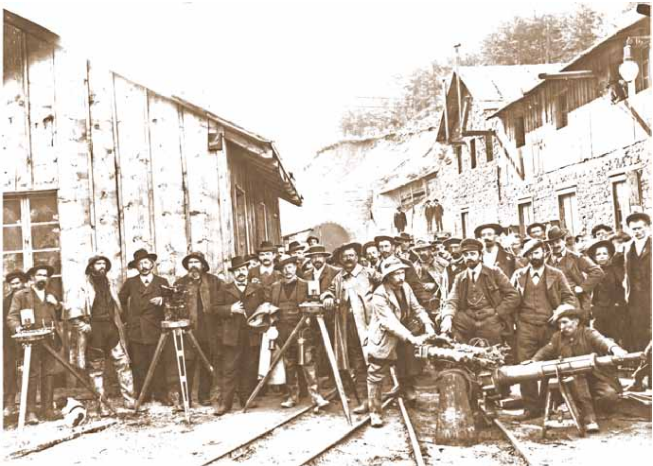
Baupersonal in Preda um 1902 (Foto: RhB)
